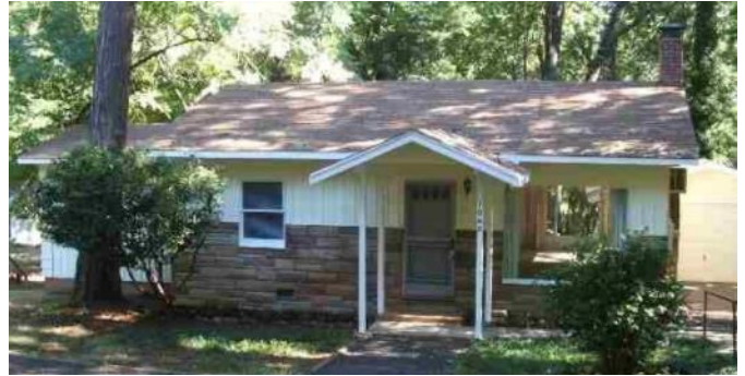
Figure 1. Street view of the original home in 2006
