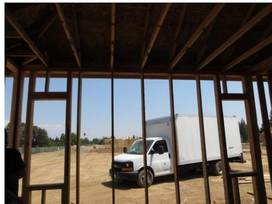
*2x6 framing lined up with roof trusses*
